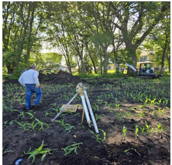
CD44 Spur 6 priority tile repair project
