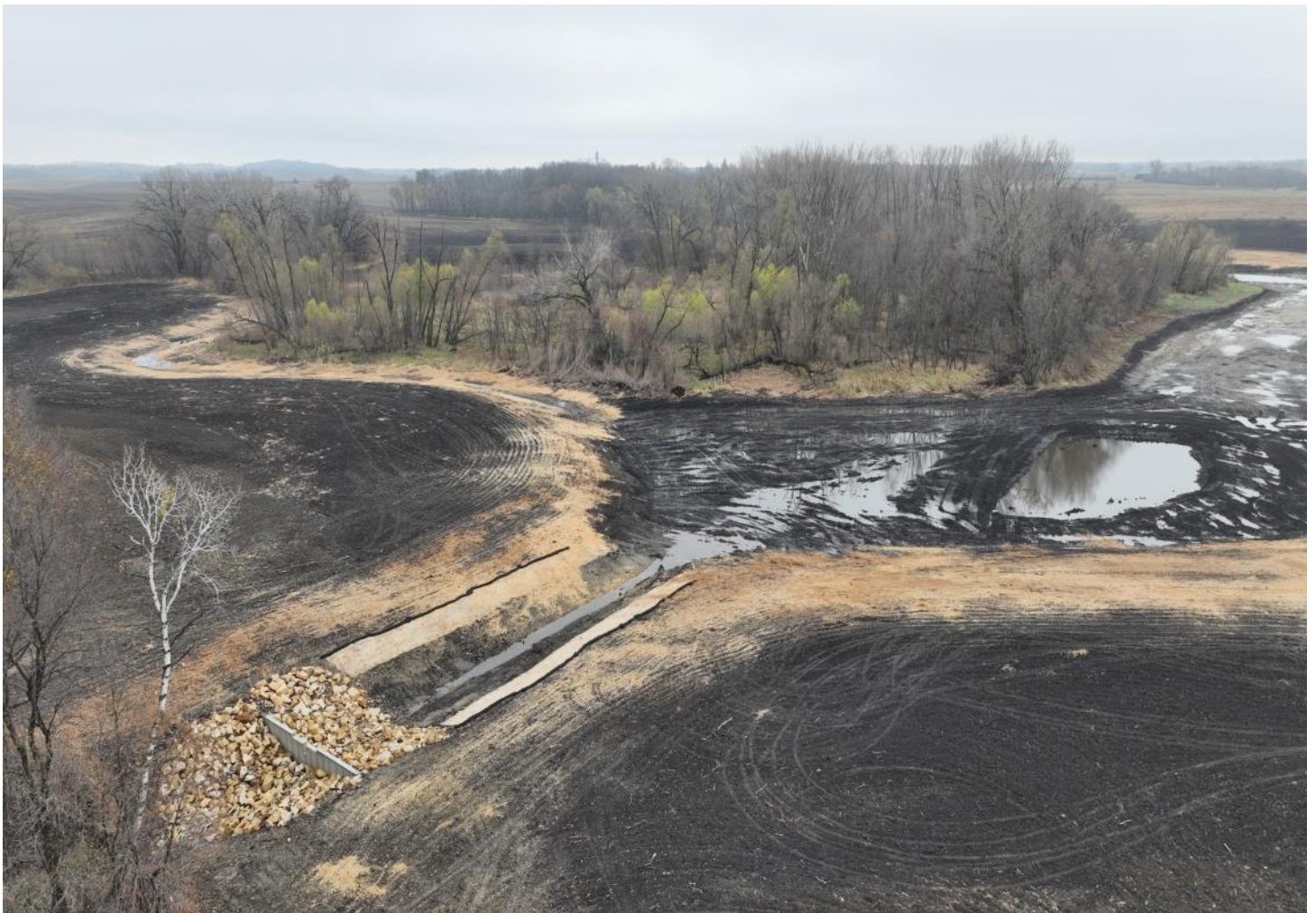
Patterson Storage Project Weir and Storage Area in the Fall of 2024
