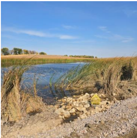
Outlet Structure & Existing Wetland
