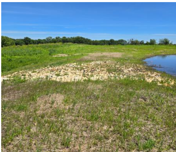
Berm & Rock Weir
