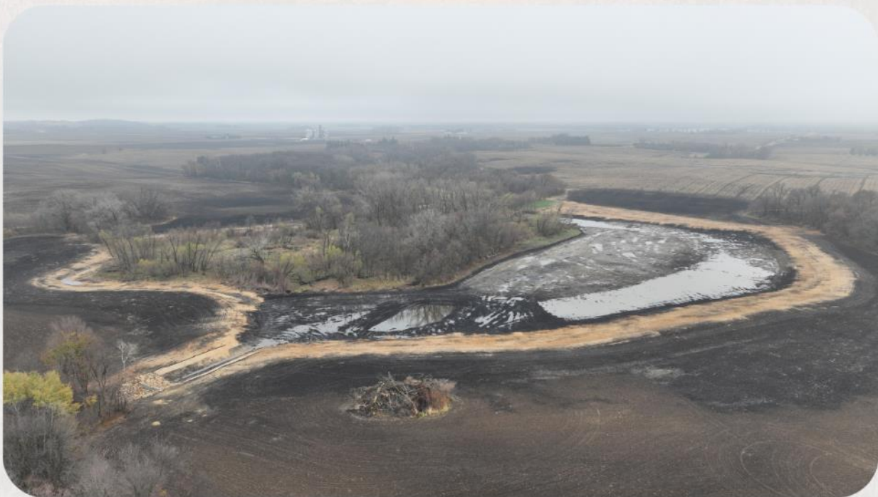
Patterson Water Storage Project after construction was completed in 2024
