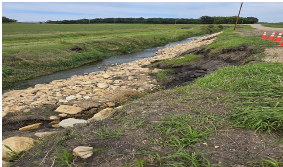
CD23 slough repair
