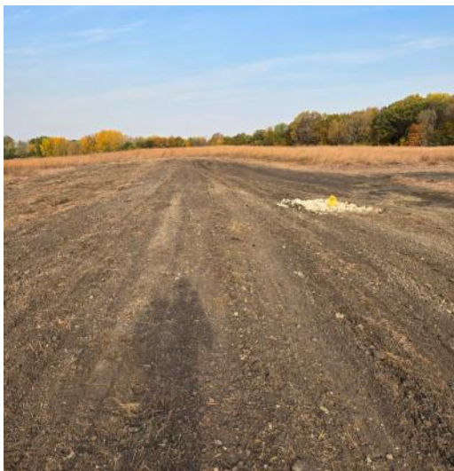
Berm & Outlet Structure
