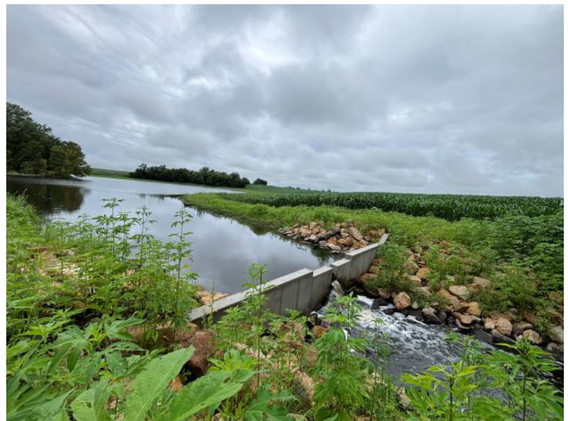
Below photo: a snapshot of the water storage project completed on the Beckel Family property in Washington Township.
