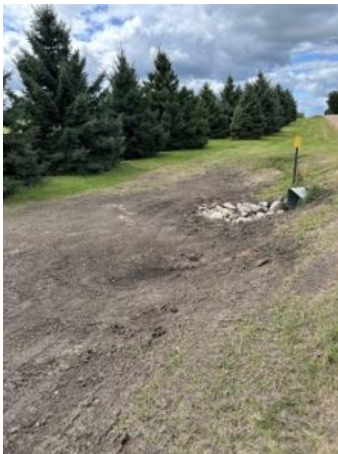
End of the repaired tile system.
