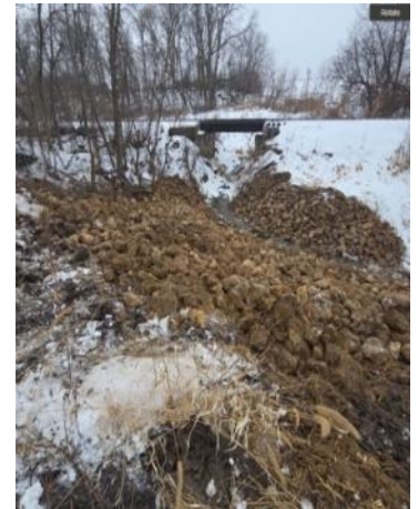
Bank repair near one of the railroad crossings.
