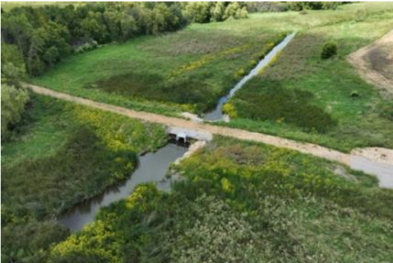
Top Left: outlet structure on CD 15.
